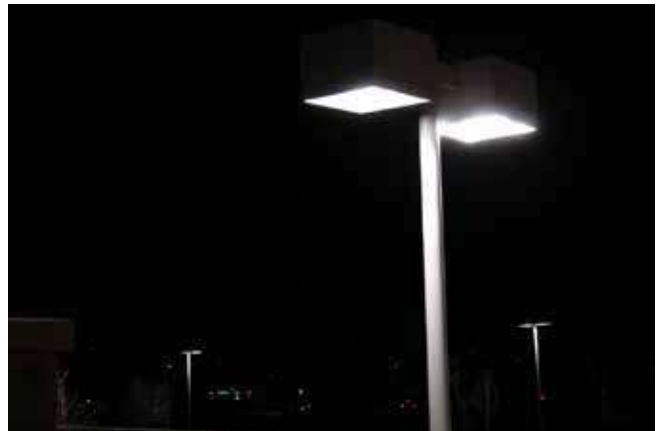
Whiter, brighter lighting should be used for accentuating entrances and pedestrian circulation.
