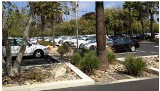
Parking lot with stormwater planters.
