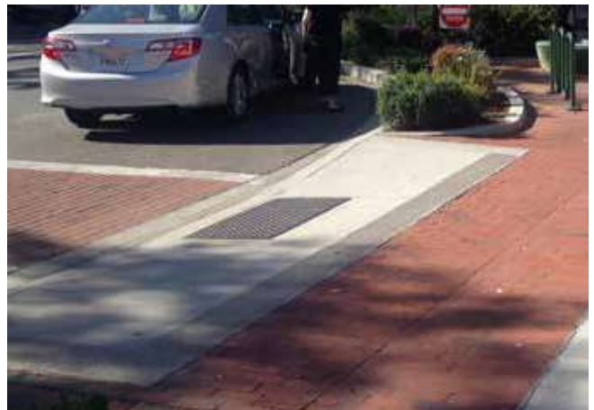
Apply paving to all corners and crosswalks to continue a "brick look."
