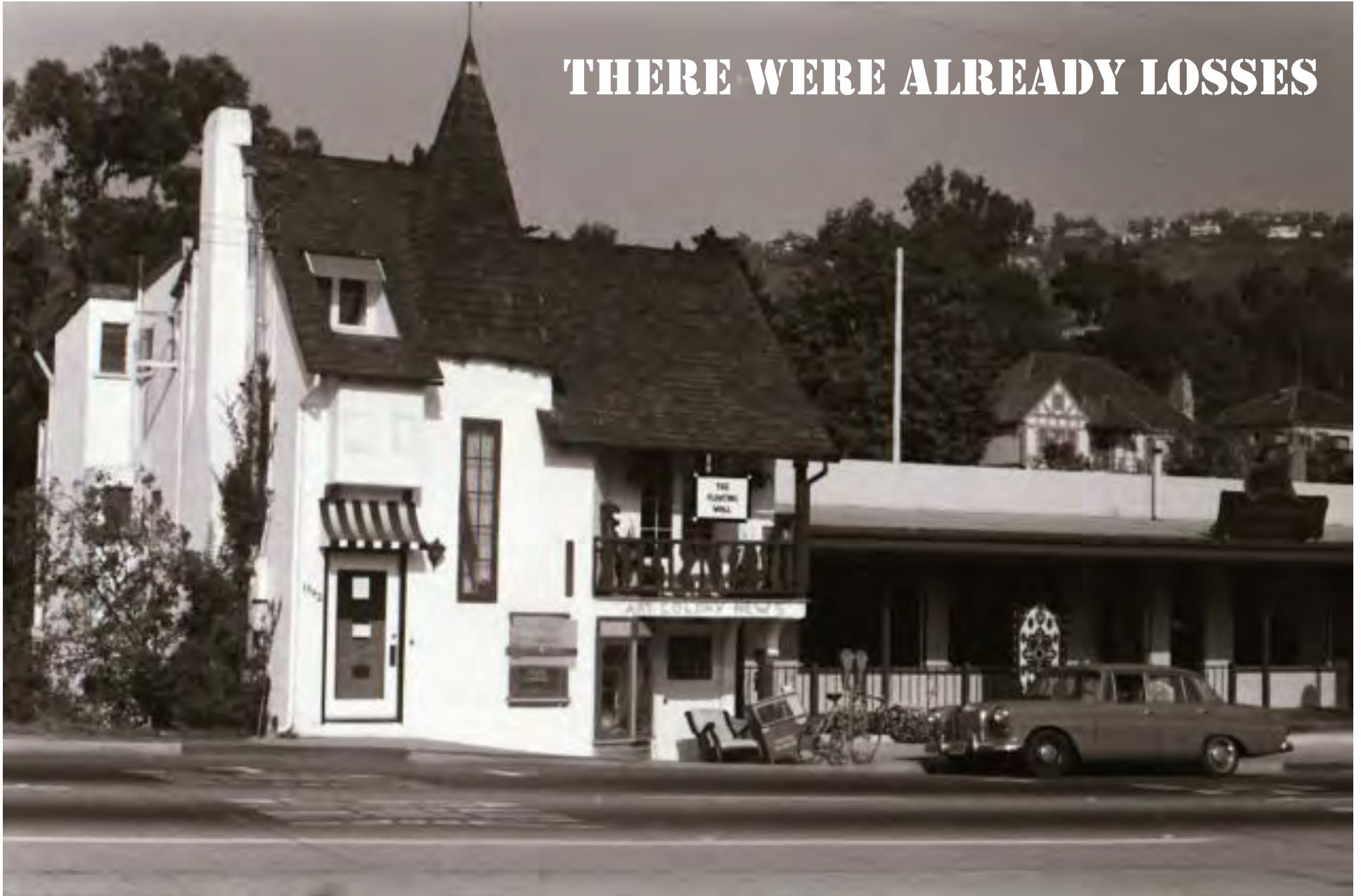
Between Calliope and Bluebird--demolished early 1970s
